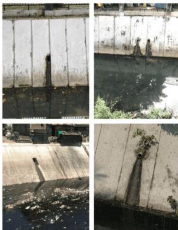
Figure 2. Household Water Lines from the Residential Area (Source: Personal Documentation, 2021)
