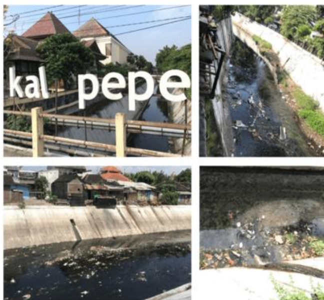
Figure 1. The Condition of Pepe River Polluted by Household Waste (Source: Personal Documentation, 2021)
